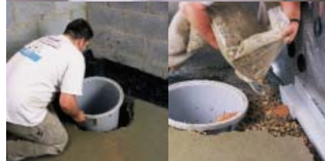
Fitting the Supersump™
